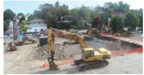
Excavation began in the summer of 2006.
