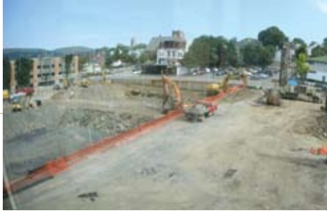
Work on the foundation continued through the summer and fall of 2006.
