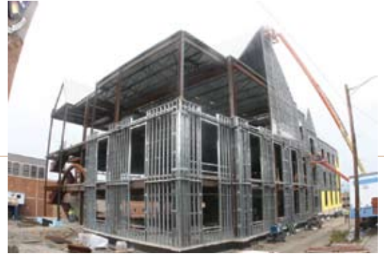
The building began to take shape with structural steel erection.
